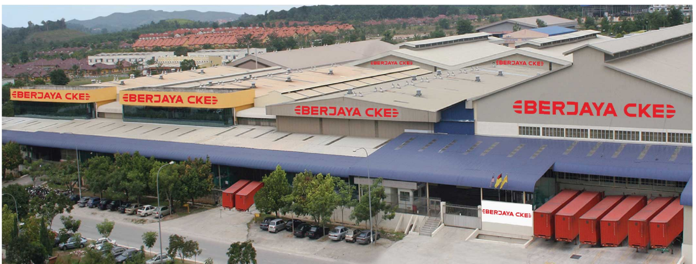
Manufacturing Plant In Negeri Sembilan, Malaysia
